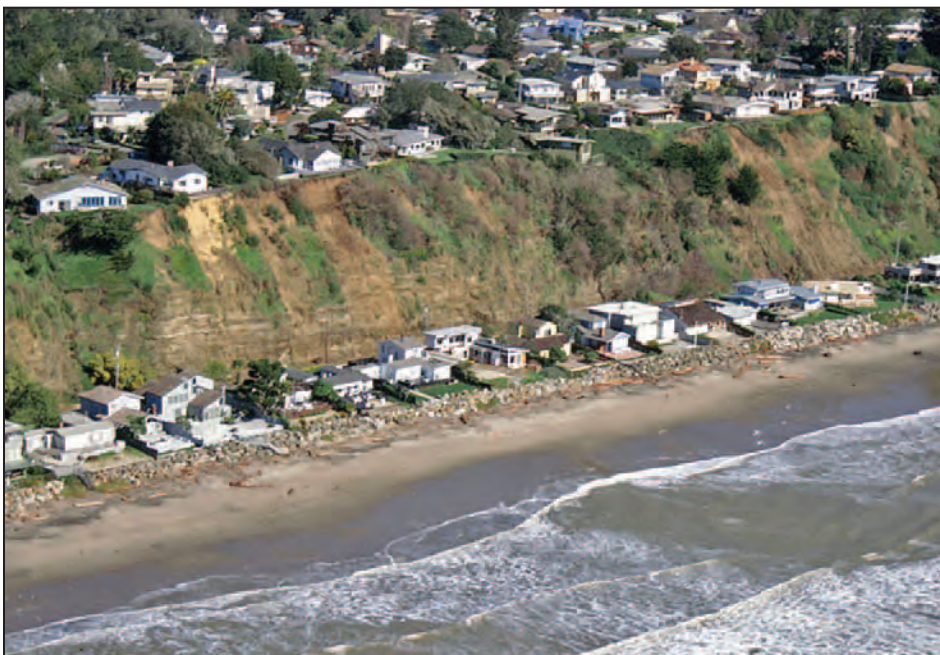
Figure 4-22. Coastal building site in Aptos, CA, provides an example of a coastal building site subject to multiple hazards
