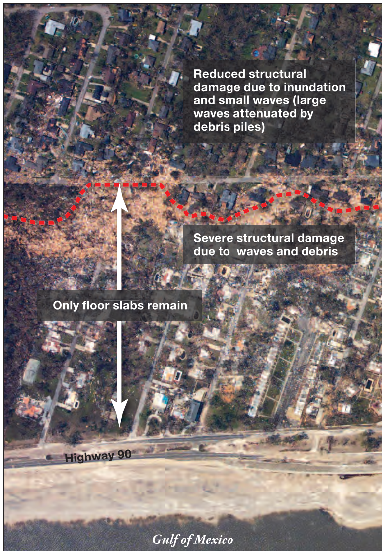
Figure 3-29. Debris generated by destroyed buildings at Pass Christian, MS (Hurricane Katrina, 2005)
