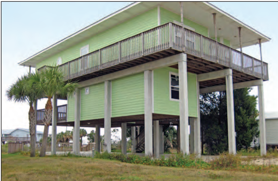
Figure 2-23. Above-grade enclosure (Perry, FL)
