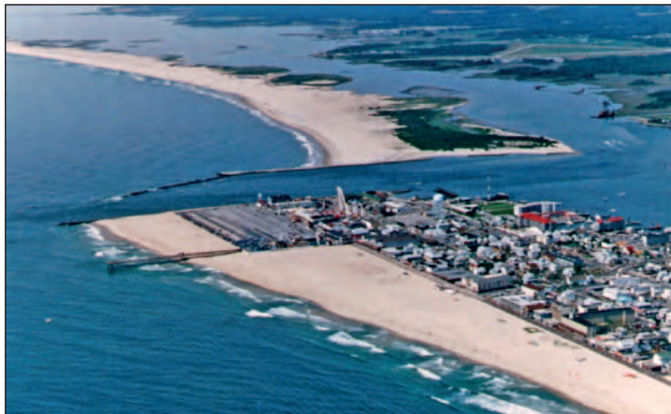
Figure 3-41. Ocean City Inlet, MD, was opened by a hurricane in 1933 and stabilized by jetties in 1934–35 that have resulted in extreme shoreline offset and downdrift erosion (1992 photograph)
