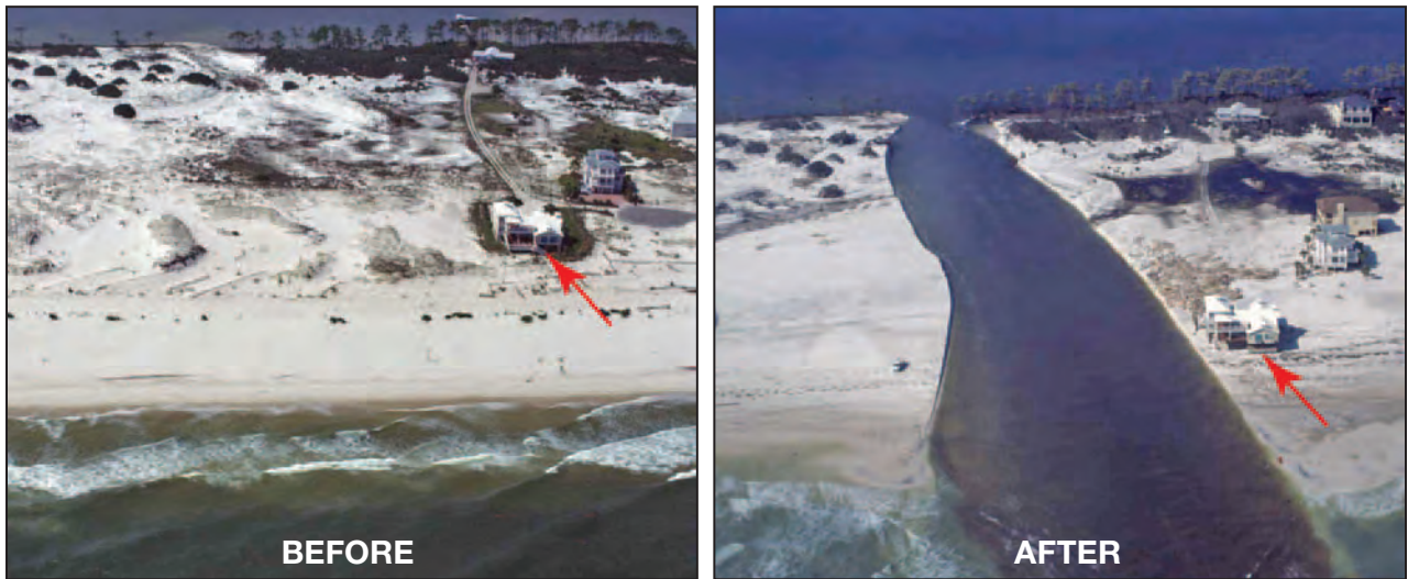
Figure 3-39. Breach through barrier island at Pine Beach, AL, before Hurricane Ivan (2001) and after (2004) SOURCE: USGS
