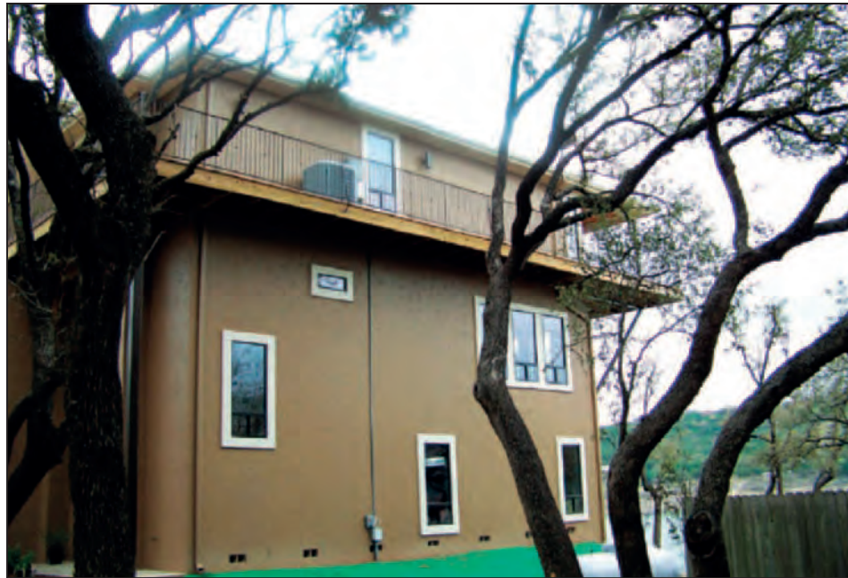
Figure 2-24. Two-story enclosure SOURCE: FEMA P-499 2010
