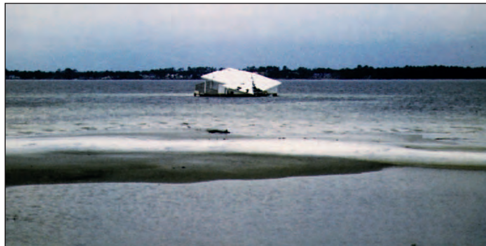
Figure 3-22. This house, located in an area of channeled flow near that shown in Figure 3-20, was undermined, washed into the bay behind the barrier island, and became a threat to navigation
